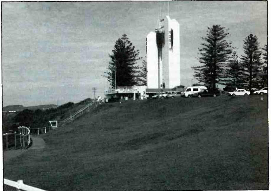
Here's the headquarters of the world's first all-emergencies volunteer communications center operated by Air Sea Rescue at Point Danger in Australia. This photo was taken by Bill Pittman, KC4YIH. Antennas are located atop the large tower as well as atop the command center at left of the tower.
